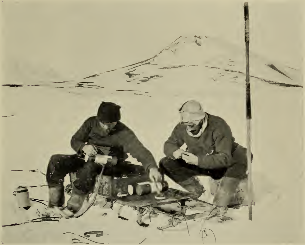
FITTING EXPLOSIVE CHARGES.
