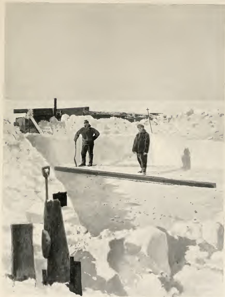
DIGGING THE FOUNDATIONS OF FRAMHEIM.
